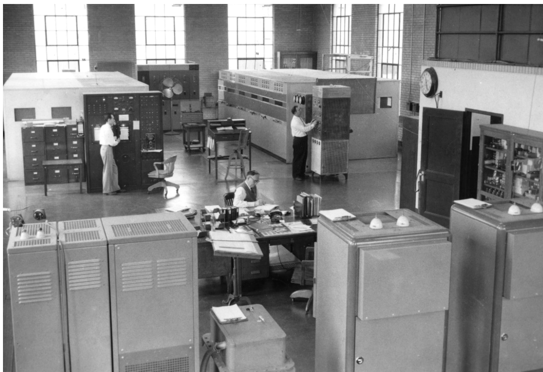
Fig. 14. Interior view of the new WWV building.
