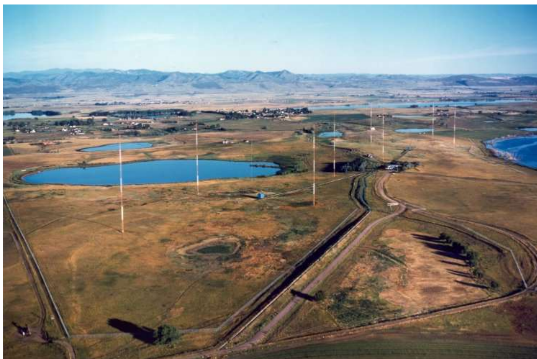
Fig. 24. Aerial view of WWVB, looking northwest.
