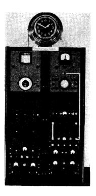
to control an oscillator, which in turn could be used to drive a clock. Because the resulting equipment, the atomic clock, is controlled by the invariable molecular system of ammonia gas, it is independent of astronomical determinations of time and unaffected by temperature, pressure, and aging.
