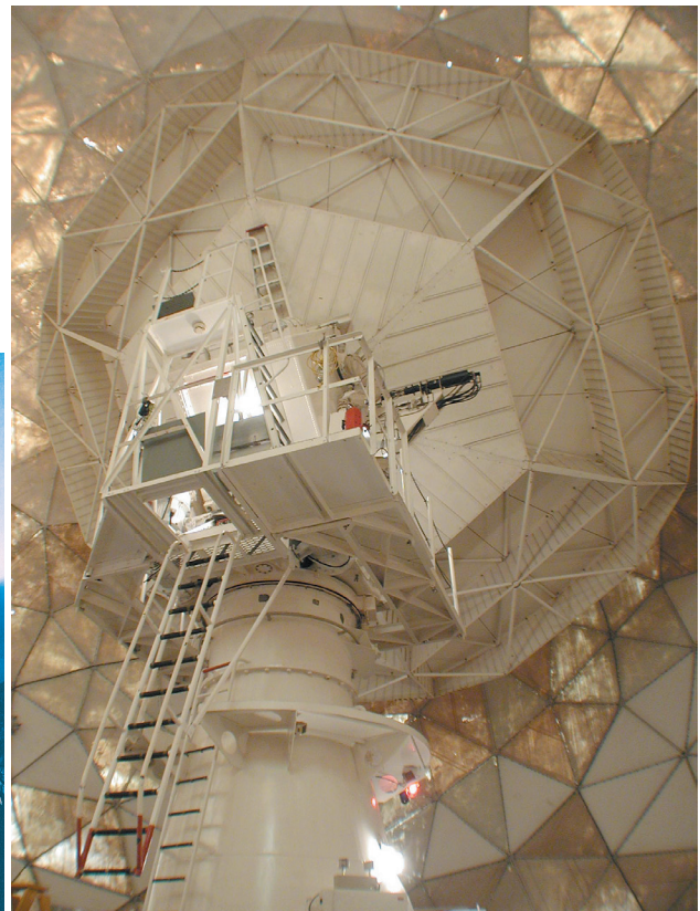
The sixty-eight-foot-diameter ALCOR radome, shown on the left, houses the forty-eight-foot-diameter antenna and its pedestal. ALCOR, which became operational at Kwajalein Atoll in 1970, was the first high-power, long-range, wideband field radar.
