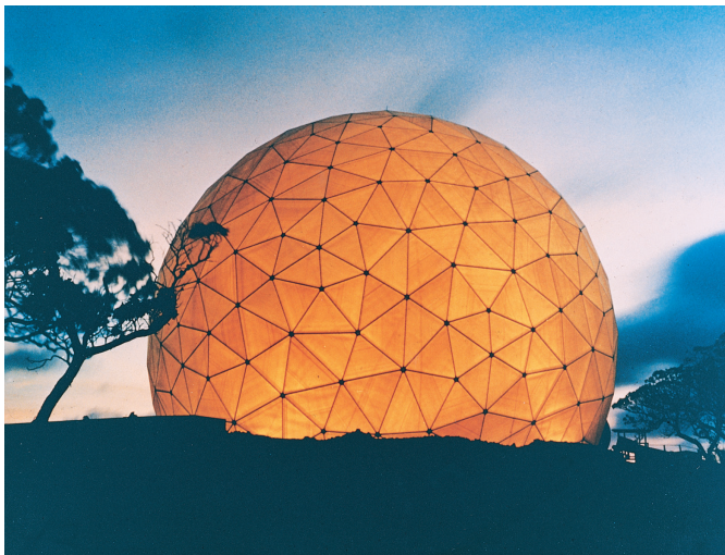
The sixty-eight-foot-diameter ALCOR radome, shown on the left, houses the forty-eight-foot-diameter antenna and its pedestal. ALCOR, which became operational at Kwajalein Atoll in 1970, was the first high-power, long-range, wideband field radar.
