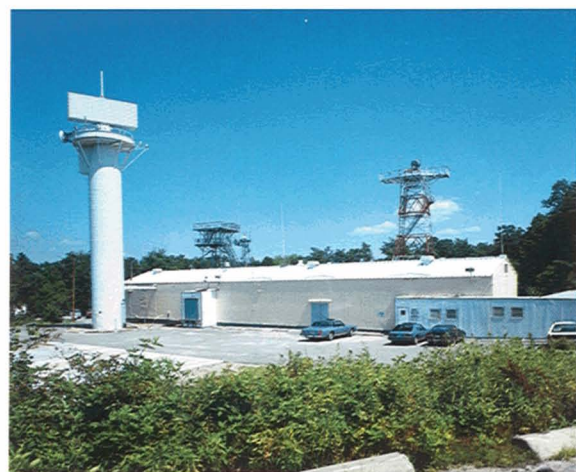
Fig. 14—The Mode-S Experimental Facility (MODSEF).
