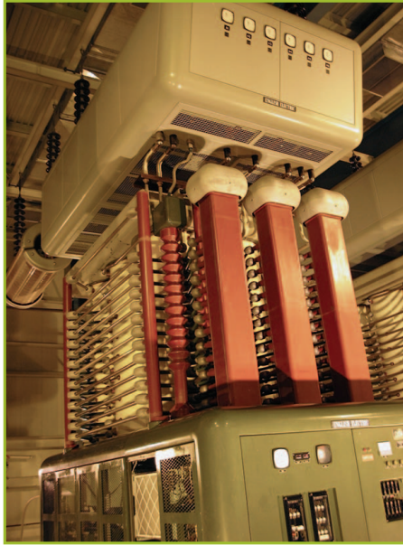
figure 1. A mercury-arc valve at the Manitoba Hydro Radisson Converter Station. (From Wikipedia, Creative Commons SA 1.0.)
