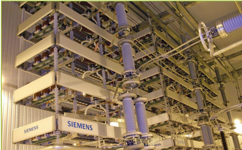
figure 5. A modern HVdc converter hall. (Image courtesy of Siemens, www.siemens.com/press .)
