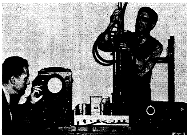
In the Bureau's study of second sound, thermal pulses generated in liquid helium II (Dewar flask, background) travel through the helium as second sound and are detected by a temperature-sensitive element, amplified, and placed on the screen of the oscilloscope.
