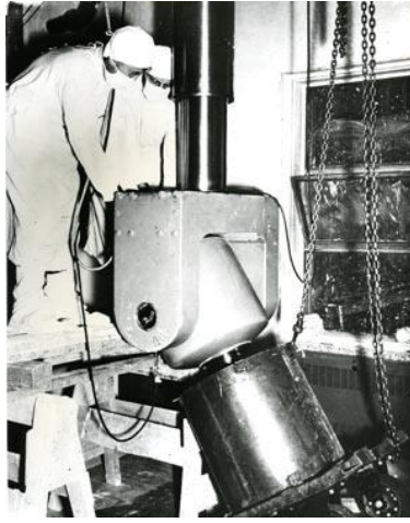
Installation of the Cobalt-60 unit in the G Wing of the University Hospital [Credit: University Archives, Harold Johns Collection]
