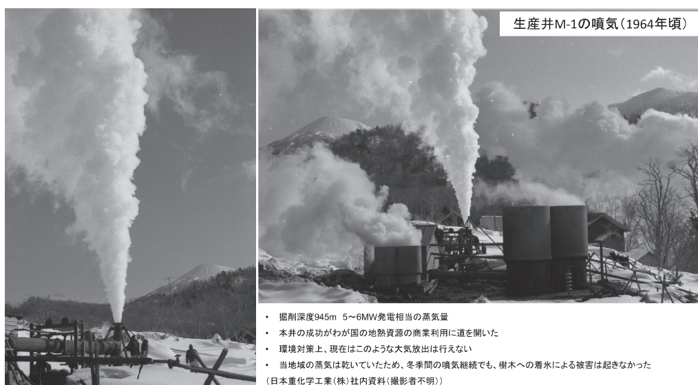
Fig.8 Steam discharge from well M-1.
