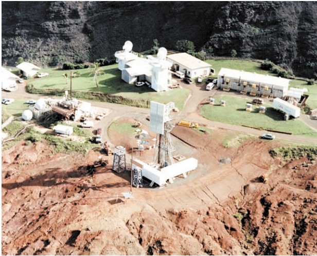
FIGURE 20. The Mountaintop radar under construction at Makaha Ridge, Kauai, Hawaii.
