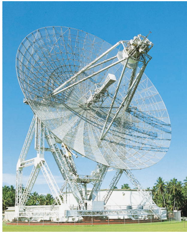
FIGURE 8. The VHF/UHF ALTAIR radar on Roi-Namur Island, Kwajalein Atoll, Marshall Islands. ALTAIR is a prime sensor for satellite tracking as well as for support of ballistic missile tests. After ALTAIR became an operational radar the UHF subsystems of the TRADEX radar were replaced by S-band subsystems.
