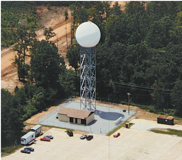
FIGURE 21. Microwave test-bed radar at the Memphis, Tennessee, airport. This radar allows airport controllers to characterize microburst phenomena in a variety of environments and climatologies.
