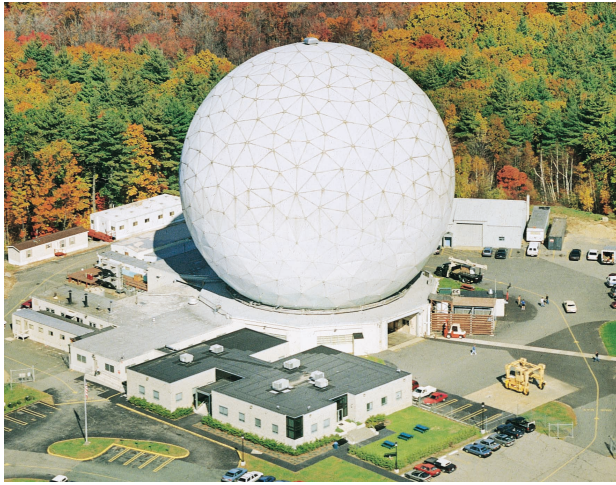
FIGURE 12. The Haystack Hill facility in Tyngsboro, Massachusetts. The large antenna within the radome has been a fertile source of advances in radio astronomy, radar astronomy, satellite imaging out to geostationary-orbit altitudes, and characterization of orbital debris.
