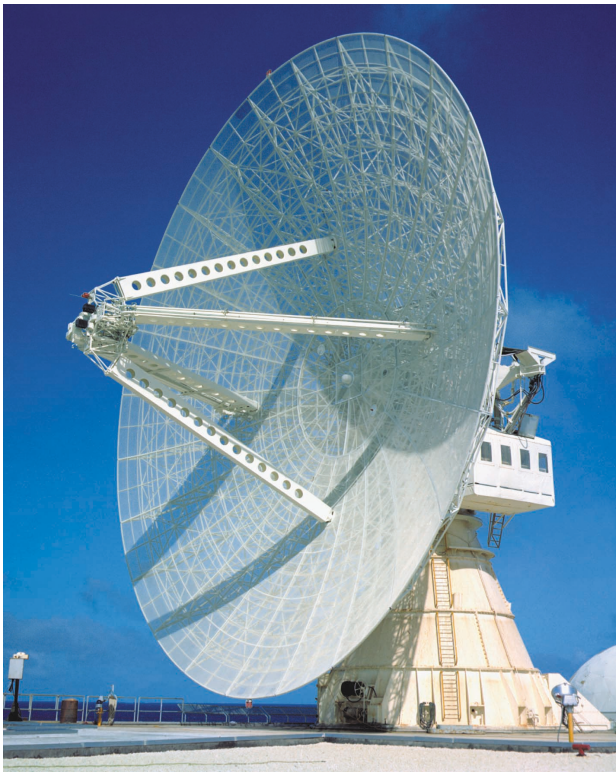
FIGURE 7. The UHF/L-band TRADEX radar on Roi-Namur Island, Kwajalein Atoll, Marshall Islands. This sensor combined outstanding performance capability with great flexibility in transmitted waveforms, tracking, and data recording.
