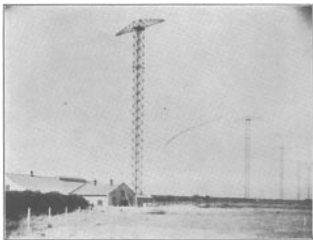
Fig. 4. Bodmin beam station. South African masts.
