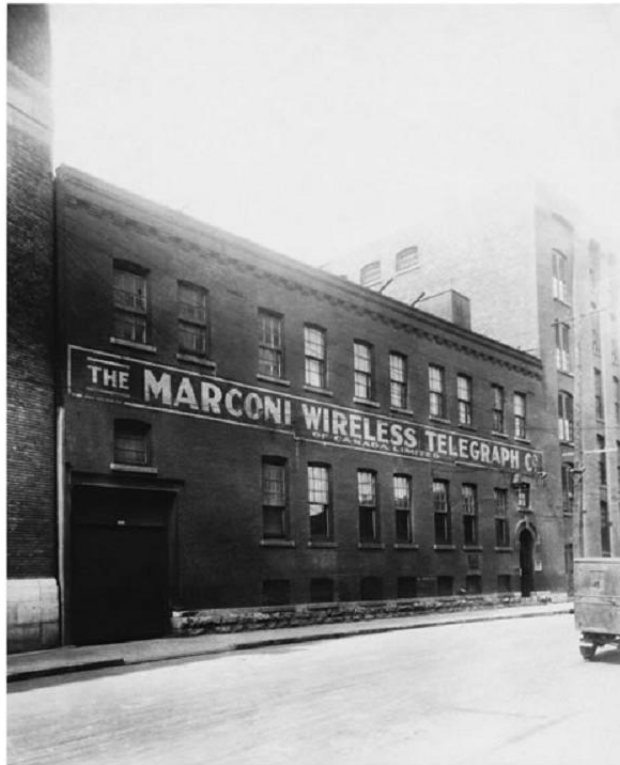
The Marconi Wireless Telegraph building in Montreal where the experimental station XWA was broadcasting.
