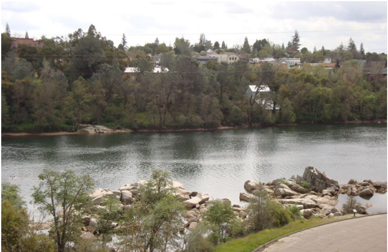
Folsom Power Houses (upper and lower) as seen from across the River
