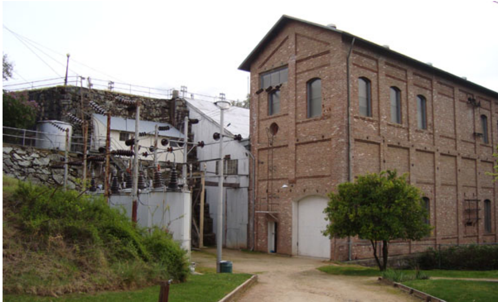
3rd Generation Transformers are located outside. (left side of photo)(800v, 60k. & 100kv)
