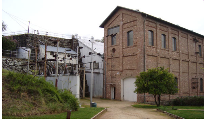
The Folsom Power House and transformers. Folsom, California (Notice the round port on the 2nd floor which allowed for the original Stanley air-cooled transformers )
