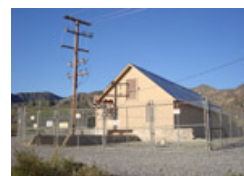
Redlands Mill Creek 1 powerhouse Redlands, CA 1893
