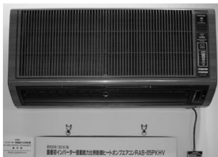
Indoor unit of the residential inverter air conditioner launched in December 1981
