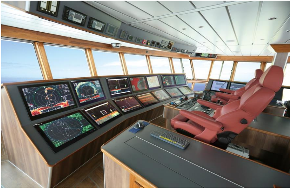
Fig. 3 A monitor panel in a bridge, in which three fishfinders and two scanning sonars are incorporated among all fourteen monitors.
