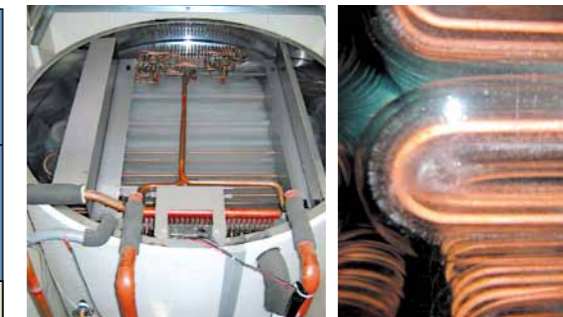
Overall appearance (on the left) and inside (on the right) of ice thermal storage tank
