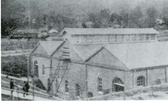
Fig. 1 Phase 1 Keage Power Station.
