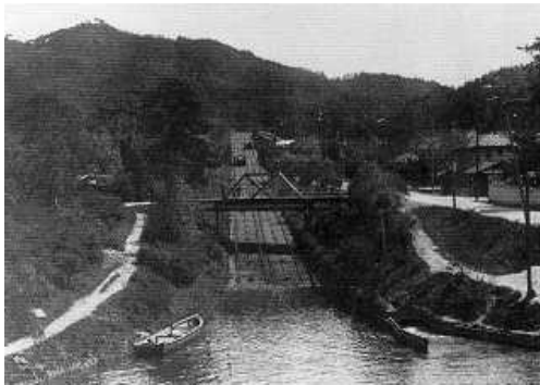
Fig. 5 Incline tracks built in the Keage Power Station
