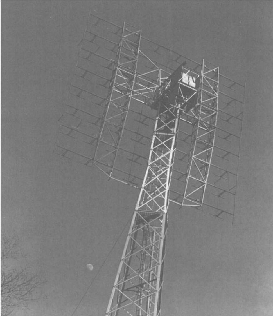
Figure 1. The "bedspring" mast antenna, U.S. Army Signal Corps, Ft. Monmouth, New Jersey, used by Lt. Col. John H. DeWitt, Jr., to bounce radar echoes off the Moon on 10 January 1946. Two antennas from SCR-271 stationary radars were positioned side by side to form a 32-dipole array aerial and were mounted on a 100-ft (30-meter) tower. (Courtesy of the U.S. Army Communications-Electronics Museum, Ft. Monmouth, New Jersey.)
